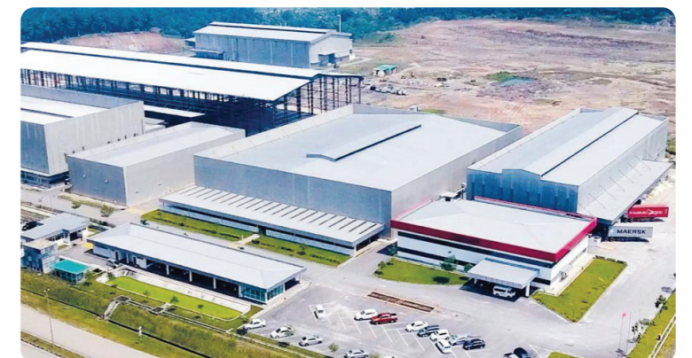
▲ Factory 38 in Kulim, Kedah, Malaysia
